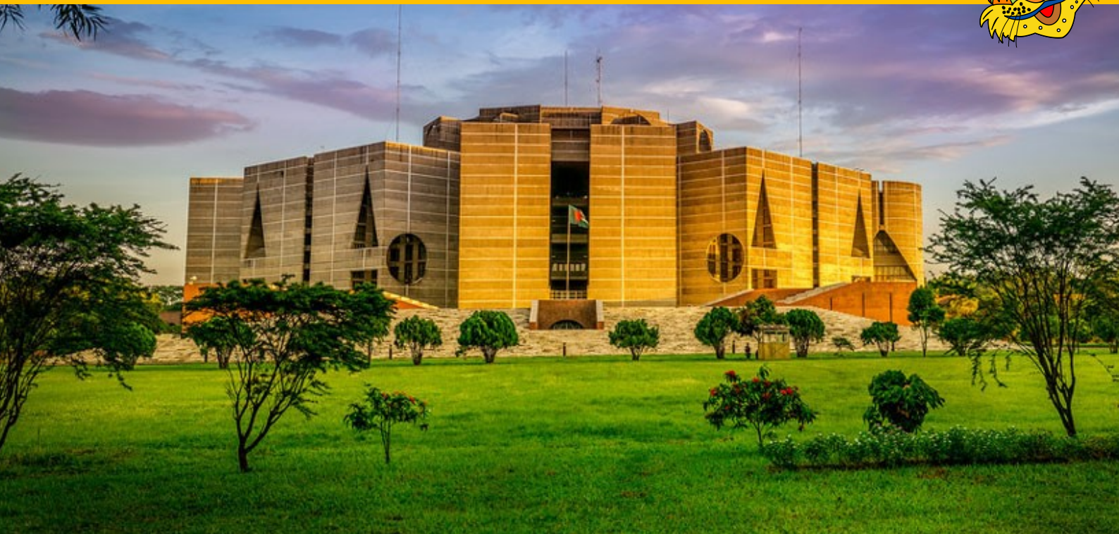
Photo: House of Parliament, an architectural masterpiece by Louis Kahn in Dhaka, capital of Bangladesh.
